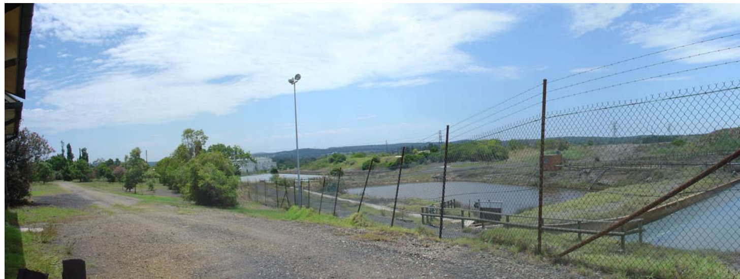
Photo 19: View north to Sugarloaf Range beyond at RL 15.00 approx.
