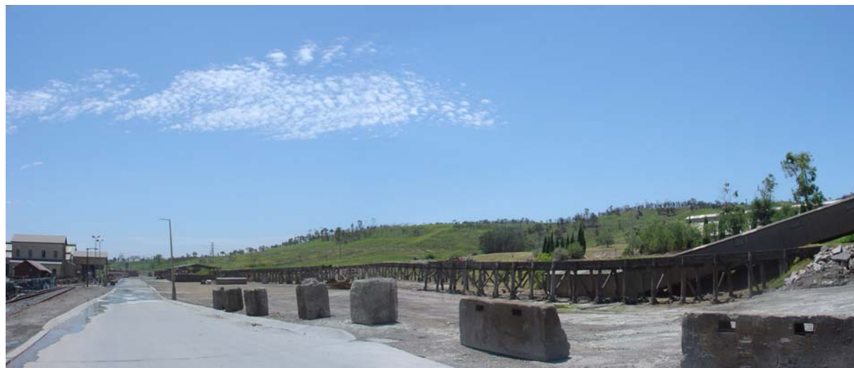
Photo 15: View north to smelter buildings at RL 25.00 approx.
