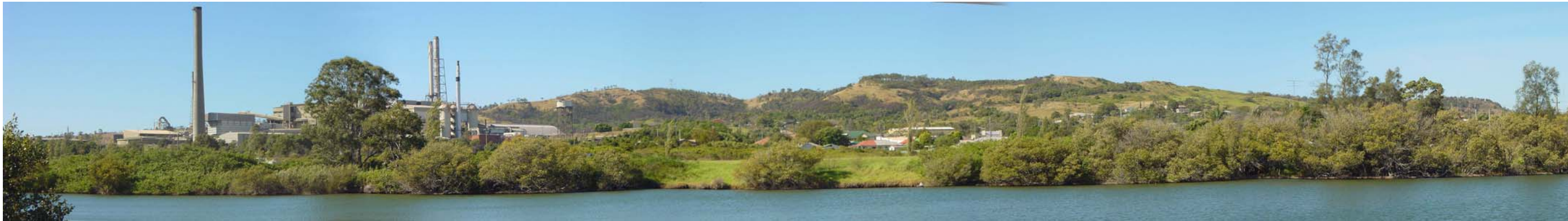
PASMINCO SMELTER BUILDINGS INCITEC BUILDING BOOLAROO RESIDENTIAL AREA HAWKINS QUARRY
